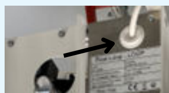
4. Cable entry via cable plug.
