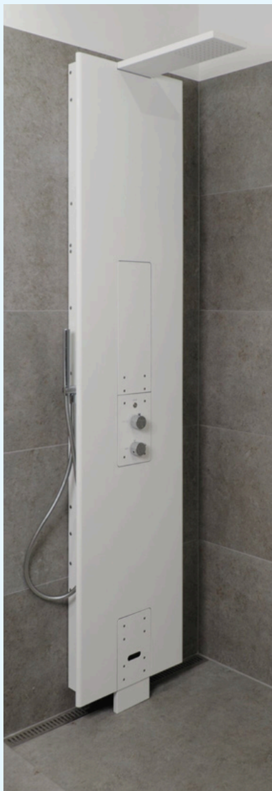
Finished linear drain.
